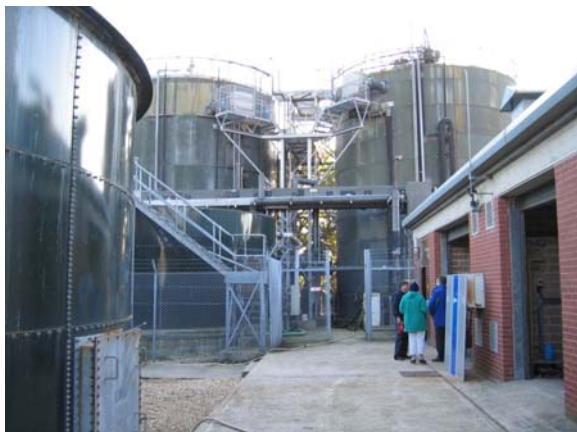
Kilminster sewage treatment works – showing anaerobic digester tanks.
