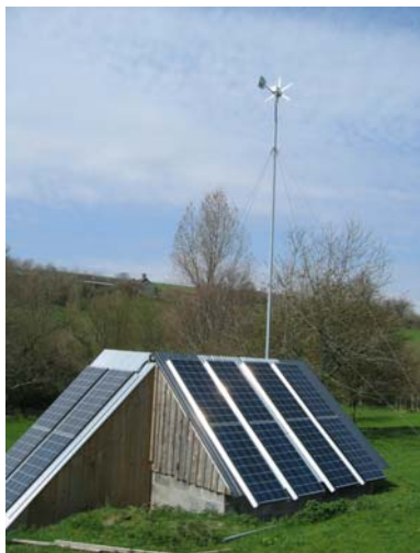
A solar power station. A purpose built shed with PV panels on the roof and a small wind generator.
