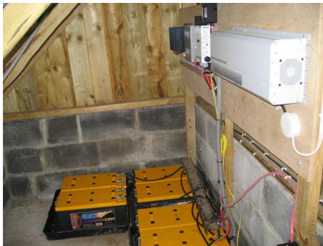
Inside the power station with the battery storage, charge controllers and sine wave inverter. The inverter changes 12 volts dc into 230 volts ac to run normal mains powered appliances.
