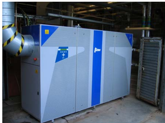
Kilminster sewage treatment works – showing gas turbine CHP. To give scale, the cabinet shown above is 2 m high x 3.5 m long x 0.75 m deep.
