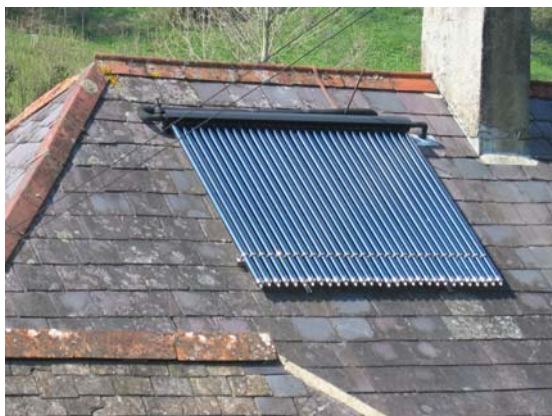
A professionally installed evacuated tube solar hot water heater that provides excess domestic hot water in the summer. The system is oversized so supplies most of the winter demand as well.
