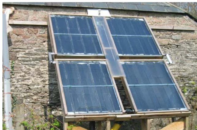
A homemade flat plate hot water collector using a design supplied by the Centre for Alternative Technology (CAT). The hot water is used to run the central heating system.
