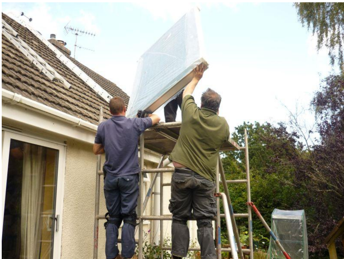
Solar panels being installed as part of TTT's 'Solar Water Heater Challenge'.
