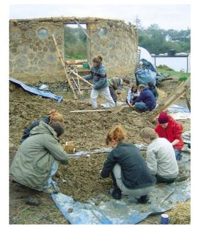
up the skills involved very quickly, and the wall contains some beautiful stonework. Plinths mortared together with lime were also built, to support the main structural timberwork.
